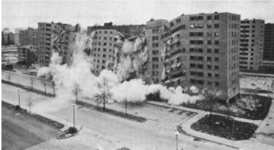
The demolition of Pruitt-Igoe, in St. Louis, MO, 1972
